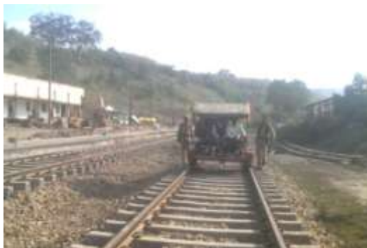
Railway engineers are seen conducting the Motor Trolley test driving in Lumding-Silchar GC Section before rolling of Diesel Engine
